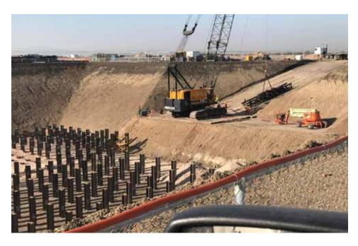
put into the ground. The design capacity of the piles was 135 tons in compression and 60 tons in tension, using HP 14x73 piles with a 70 feet embedment depth. This was one of the first jobs in this region to use steel piles instead of concrete.
